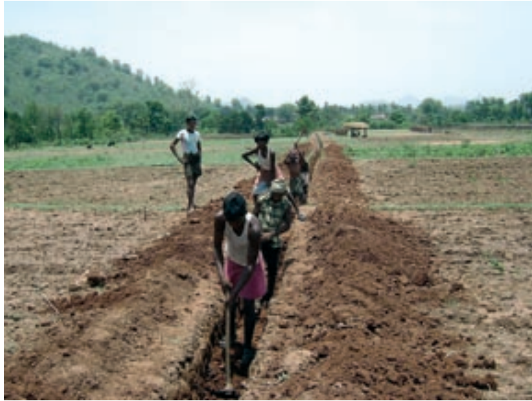
Collective action for a better future: construction of an irrigation canal
