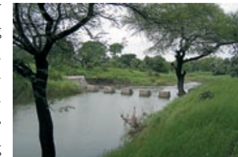
Check dam construction for promoting groundwater recharge and irrigation
